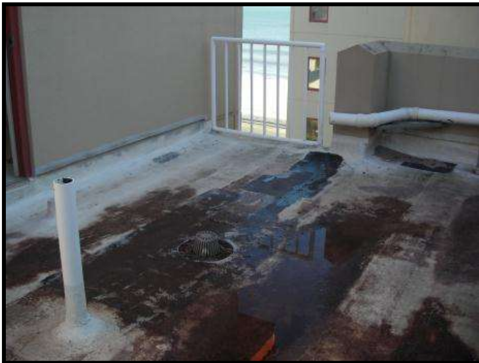
Photo 8: View of one of the low-sloped upper roof.
